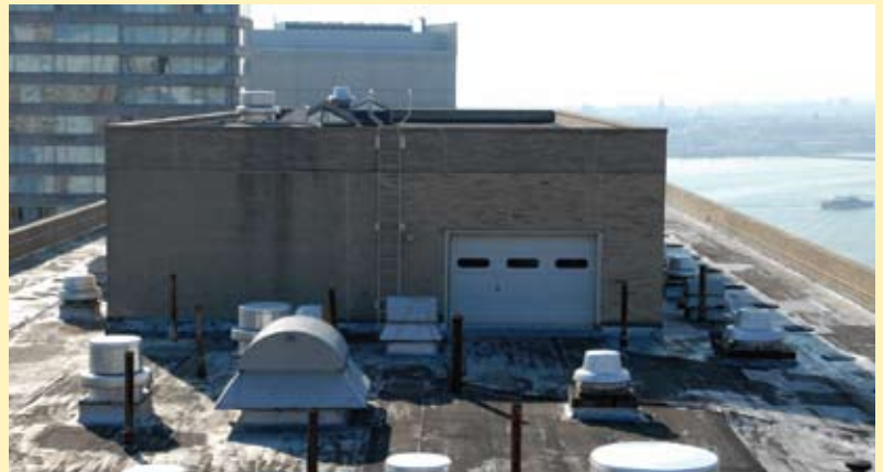
Kips Bay bulkhead: a board on top of the situation.
